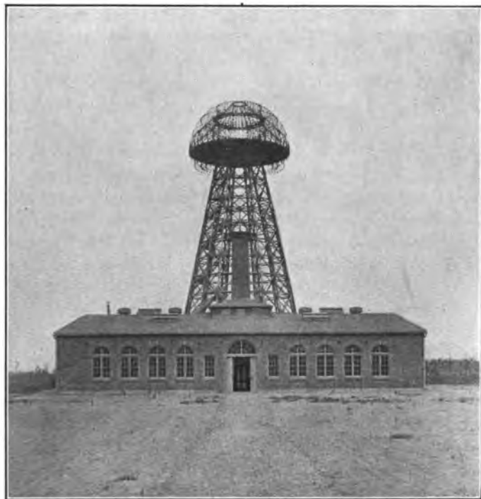
FIG. 155.—Tesla world power plant (experimental station).
