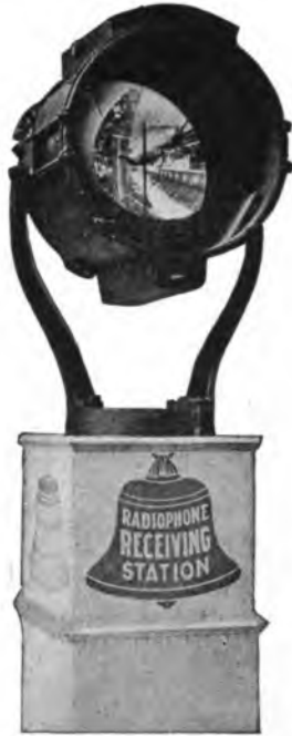
FIG. 136.—Powerful searchlight arranged to transmit speech over a beam of light.
