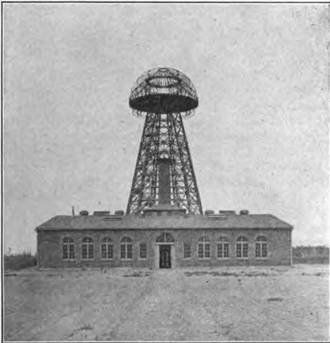
FIG. 155.—Tesla world power plant (experimental station).
