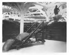
Fig. 1. Brown Portable Elevator Stacking Rough Rice in Sacks
