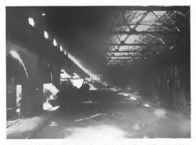
Fig. 10. Charging Side of Open Hearth Plant showing Motor-Operated Charging Machine
