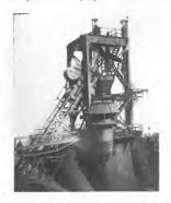
Fig. 6. Top Rigging of Blast Furnace showing a Skip Car about to Dump into the Upper Bell
