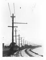
Fig. 5. Strain Insulator as a pull-off installed on a curve on a 6600 Volt Catenary construction
