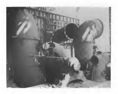
Fig. 7. Installing Water Wheels in Station No. 3
