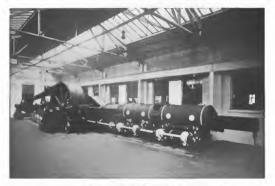
500 H. P. Gas Engine Built by the Sargent Engine Co., Driving 300 Kw, Direct Current Generator
