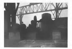
Fig. 2. 736 Kw. Induction Furnace, Showing Tilting Mechanism (Copyrighted by American Electric Furnace Co., reproduced by permission)
