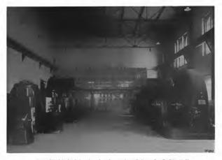
Fig. 3. Virginia St. Substation of the International Railway Co., Buffalo, N. Y. 1000 Kw. Converters with Three-Phase Air-Blast Transformers
