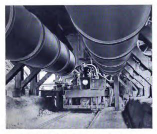
Motor-Driven Scale Car, Operating Under Ore and Limestone Pockets Illinois Steel Company (See page 3)
