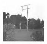
Fig. 7. Transmission Tower equipped with Link Suspension Insulators representing a 125000 volt installation
