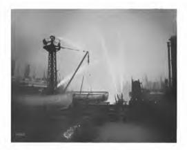
Fig. 6. Trial of Turbine Driven Pump for New York City Fire Boat
