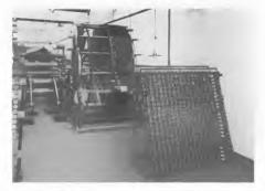
Fig. 1. Silk Warper Driven by General Electric KG 3 4 H. P. Motor
