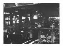
Fig. 15. A 24 in. Structural Shape Mill with Motor-Operated Traveling Tilting Tables
