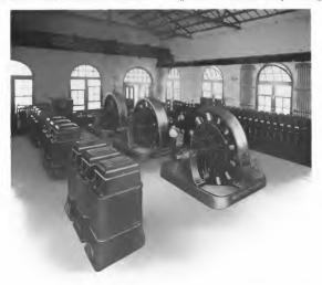
Fig. 4. Interior of the Palisade Substation of the Public Service Corporation, Newark, N. J. 1000 Kw. Converters with Single-Phase Air-Blast Transformers
