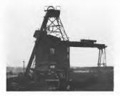
Fig. 2. Shaft House for a deep mine in the Lake Superior region with skip car about to dump and with loaded railway car under the pockets
