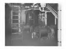
Fig. 3. Two 25 Kw. 125 Volt Curtis Steam Turbine Sets Installed on Hudson River Day Line Boat "Hendrick Hudson"
