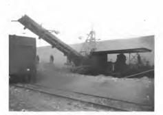
Fig. 2. Rear View of Covington Coke Extractor, Showing Controller for Ram, and Handwheel for Varying Angular Position of Ram Travel
