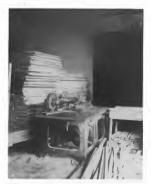
Fig. 3 Automatic Rip Saw Driven by 15 h.p. Constant Speed Motor Located In Basement
