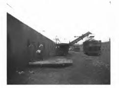
Fig. 1. Covington Coke Extractor drawing Coke from "Beehive" Oven and loading into Car. This Illustration shows arrangement of Ovens at Typical Machine Plant
