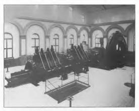
Blast Furnace Gas Engine Built by the Gas Motoren Fabrik, Nürnberg
