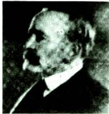
Two photographs after they had been transmitted a distance of eighteen miles by the Jenkins television apparatus.
