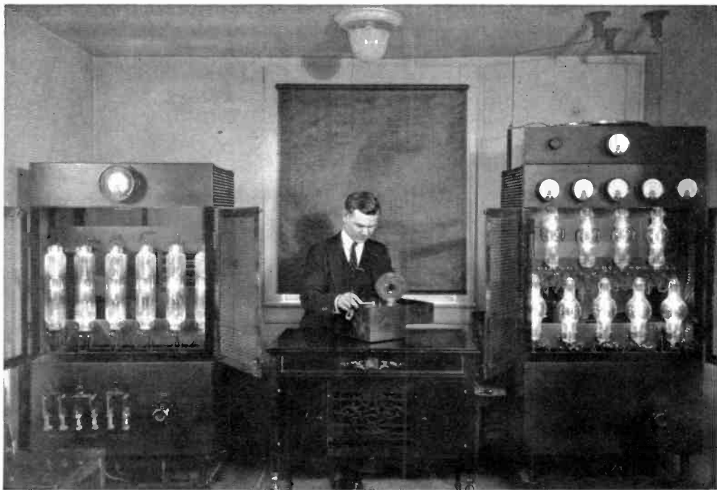
BROADCASTING TRANSMITTER AT "OLD WJZ", NEWARK, N. J.
