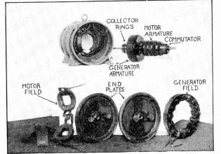
Fig. 15.—Exploded and Assembled Views of a Two-Kilowatt, Five Hundred Cycle Motor Generator Having Revolving Armature. (Courtesy of Crocker-Wheeler Company, Ampere, New Jersey.)
