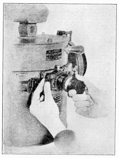
Fig. 50.—Adjustment of Arc Length.
