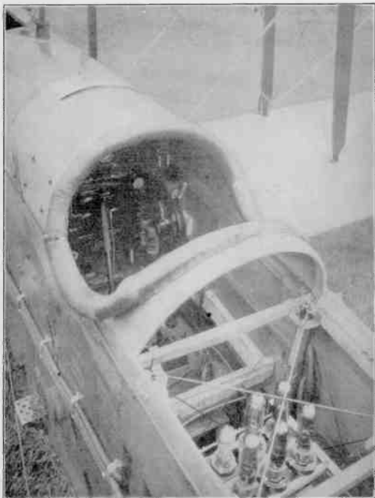
PLATE IV.—Airplane radio installation. ( Courtesy, Radio Corporation of America. )
