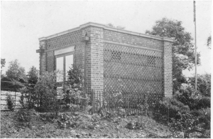
FIG. 35.—A typical form of rectifier sub-station construction which is cheap and yet pleasing to the eye.
