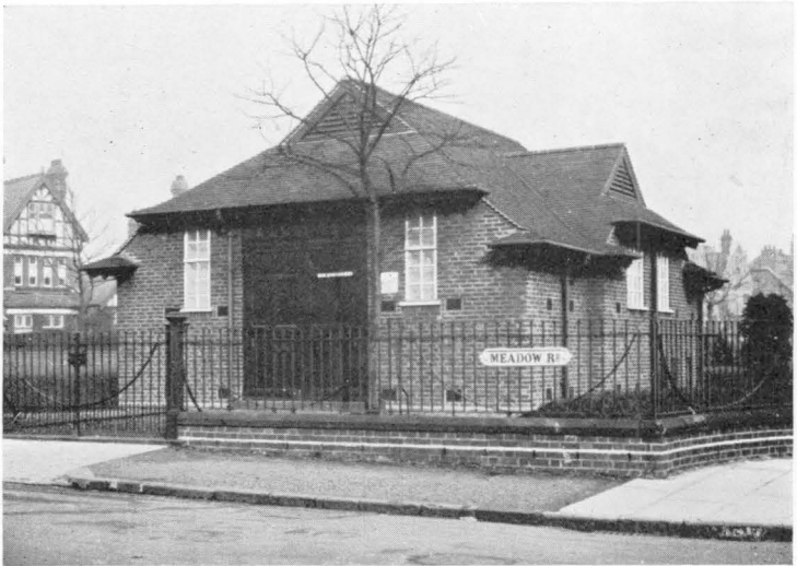
FIG. 36.—A really pleasing type of sub-station architecture.
