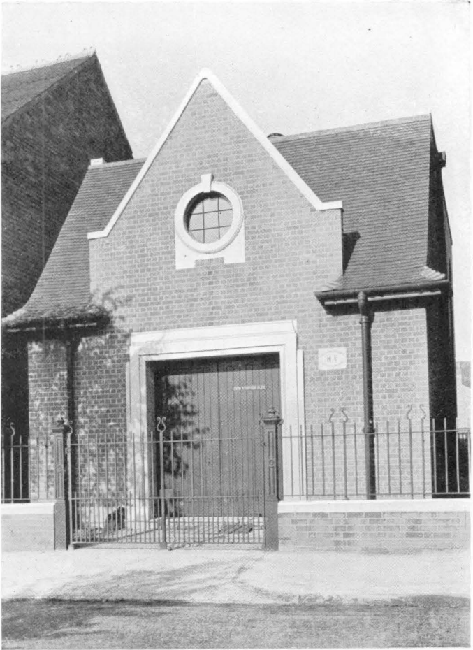
FIG. 39.—Another pleasing type of sub-station architecture.
