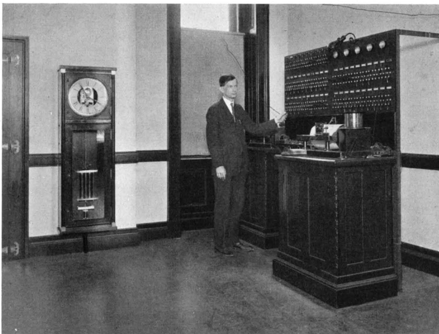
FIGURE 3. The time room at the Naval Observatory. The clock is the apparatus for sending the daily time signals, and, during the period of signaling, controls directly the broadcasting stations at Arlington, Annapolis, Key West, and San Diego, with which it is connected by wire. Connections are made through the switchboard on the right. The seconds as sent by the clock and as received by radio are recorded on the revolving sheet of paper of the chronograph on the right
