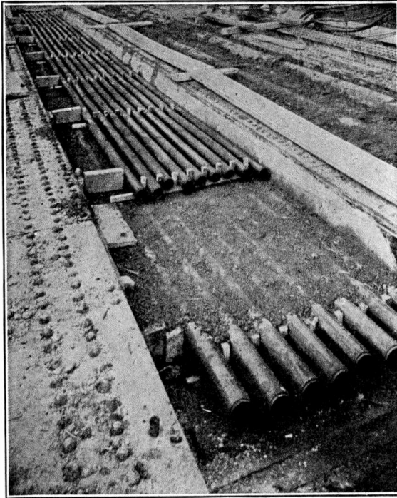
Fig. 77. Method of Laying Fibre Conduit in Trench.
