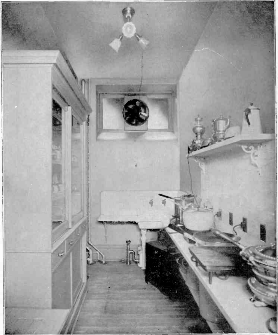
ELECTRICAL KITCHEN IN EDISON BUILDING, CHICAGO
