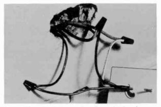
Fig. III-6. A third wire is fastened to the outlet box for grounding. Splice the wires to the "feed-in" cables with wire-nuts.
