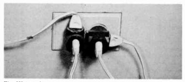
Fig. III-1. A duplex outlet trying to handle five appliances through the use of cube taps. It is hazardous and should be replaced with more outlets. cables would be a lot of work—chiseling plaster and fishing cable—especially since all five outlets are to be within a five-foot space. The answer is in *surface wiring*. As the name implies, this is wiring on the surface, or outside the wall.
