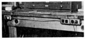
Fig. I-1 Surface-mounted utility boxes are mounted on the front of the workbench. The outlets on the right have grounding terminals, for three-prong safety plugs.
