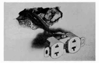
Fig. III-5. Unscrew duplex outlet and pull towards you to bring out the wires.
