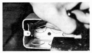
(B) Slug is then removed with pliers. Fig. 4-4. Method for removing knockouts from boxes.
