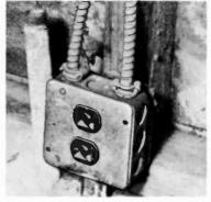
Fig. V-4. The four-inch junction at the entrance of the cable to the garage.
