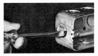
(A) A light tap on a screwdriver pushes the knockout part way out.
