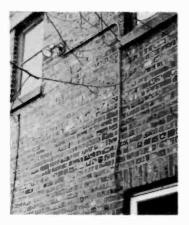
Fig. IV-1. It is important that wiring to an outside light be fully weatherproof. The use of thinwall conduit to carry the wires is a must.
