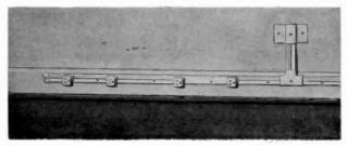
Fig. III-7. The finished surface wiring installations. Additional outlets are easy to add; they snap into place anywhere along the cable strip.
