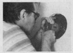
Fig. 5. Remove any insulation between the inner and outer walls and then drill through the exact center of the outer wall. The hole will be the pilot when you're working on the outside. If the wall is masonry or brick use a carbide tipped bit. A standard bit is okay for a frame construction (wood siding).
