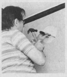
Fig. 2. If the wall is sheetrock (drywall) score the outline with a knife, a narrow chisel, or an old screwdriver, then cut all the way through and punch out the circle.
