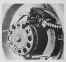
Fig. 12. Here is a close-up of the fan motor and electrical connections. BX cable comes from house wiring and connects to an electrical box mounted on the motor. Wire nuts cover the splices.
