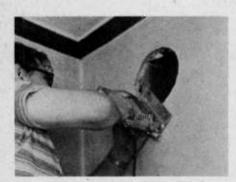
Fig. 4. If you have made a measuring error and find a stud running past the hole, don't panic. The wall will stand even if you cut through one stud. Use a saber saw to trim the stud so the cuts correspond to the circular duct pattern.
