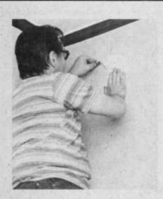
Fig. 1. Pick a location for the grille-damper, and make certain it's between two wall studs. Using the duct as a template, scribe the outline on the wall and then use a razor to cut away the wallpaper.
