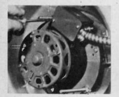
Fig. 13. After the connection has been made, the box cover is screwed in place. Now check that the fan rotates freely and the housing is secured firmly to the wall. Some weatherproofing caulking is necessary. Less than one half a cartridge from a grease-gun squirter is needed.
