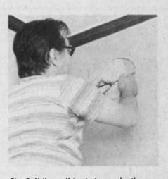
Fig. 3. If the wall is plaster, scribe the outline and then chip out the plaster until the lath is exposed. The lath can be either strips of wood, wire mesh, or plasterboard —a sheetrock-type material with a pattern of large holes into which the plaster locks when dry.
