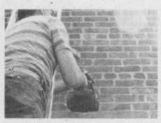
Fig. 8. The final trim is done by hand with a cold chisel and small sledge. The sheet metal duct should just slide through the hole without bends or a force fit. Chip away small bits of brick until the duct can slide in and out easily.
