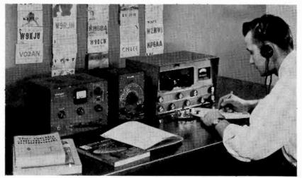
Fig. 911. Communications receiver being used in a ham station. (Allied Radio Corp.)
