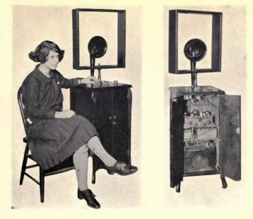
The author's "Radiotrola." This machine was built late in 1921, and is the first radio machine of its class to take on the appearance of a piece of furniture. The Radiotrola, now used in the author's home employs neither antenna nor ground, the reception being made by the loop shown in the engraving. The music, as well as entertainment, from WJZ, Newark, N. J., although twelve miles distant, comes in so loud that the sounds can be heard all over the apartment.
