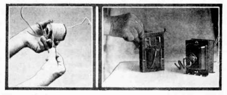
FIG. 6A and 6B—Left, rewinding a power transformer. Right, first replacing the laminations and finally, the completed instrument, looking as good as new.
