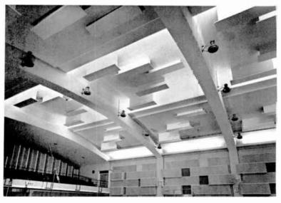
Fig. C/17. Maida Vale Studio 1. Excellent view of ceiling showing variation in size and shape of scattering elements. Note also boxes on side walls which act as acoustic absorbers and diffusers, with special treatment of wall behind small balcony where audience is accommodated.
