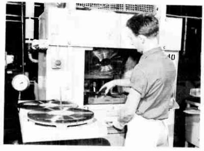
Fig. R/13. Pressing the final record.
