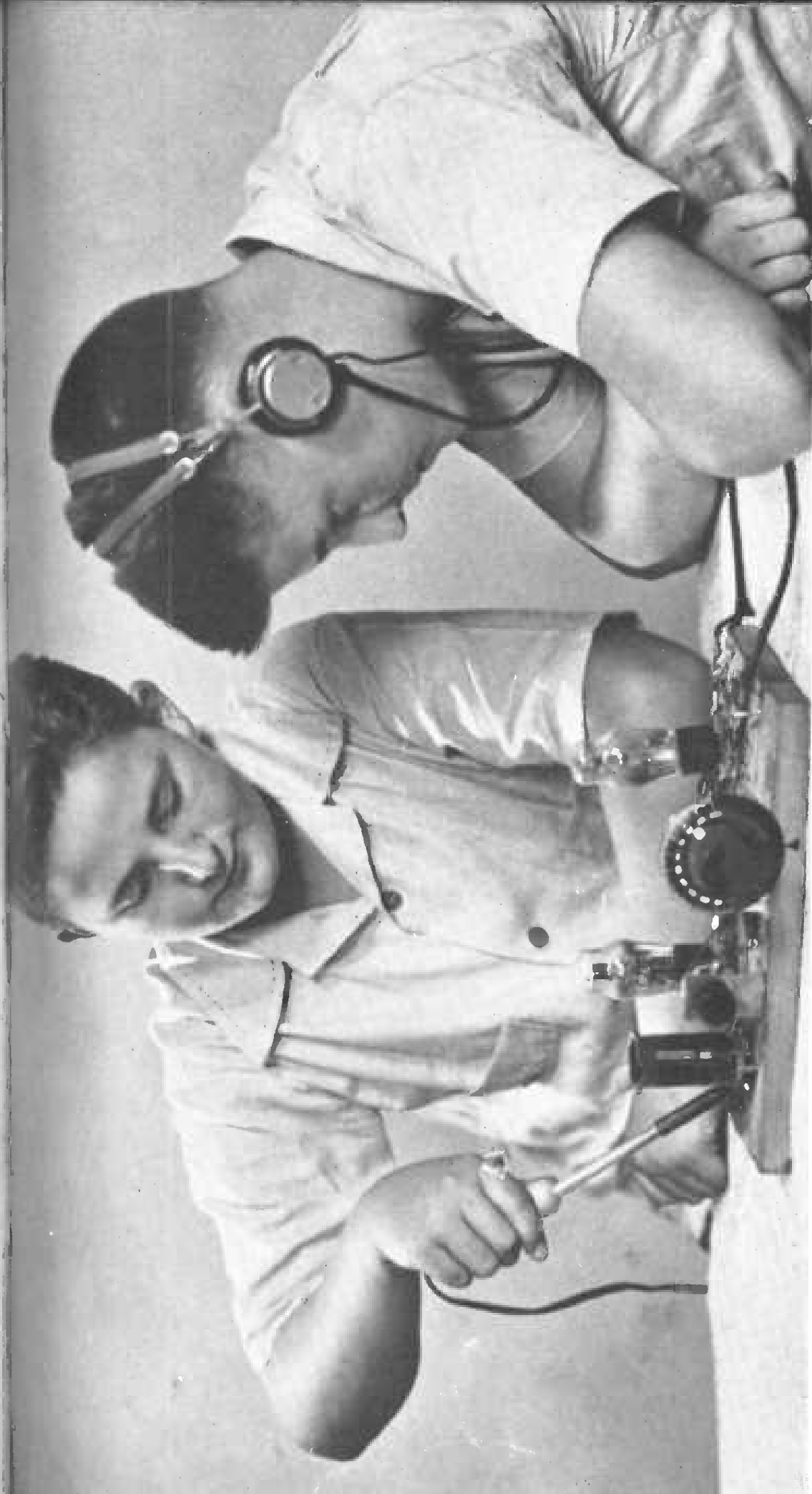
Soldering plays an important part in the successful building of radio apparatus. Hold the hot iron firmly against the connection until the solder spreads out or "sweats" into the connection.
