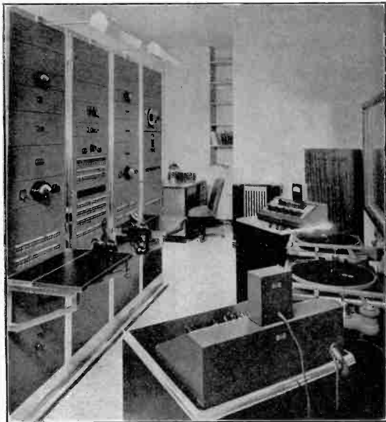
FIG. 1 —Radio broadcasting station showing speech input equipment and control switchboard. (Courtesy Western Electric Co.)
