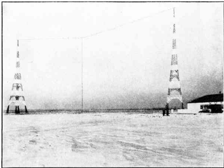
FIG. 2 —General view of antenna system of a large transmitting station showing two steel towers each 385 feet high and the transmitter house off to one side. (Courtesy Western Electric Co.)
