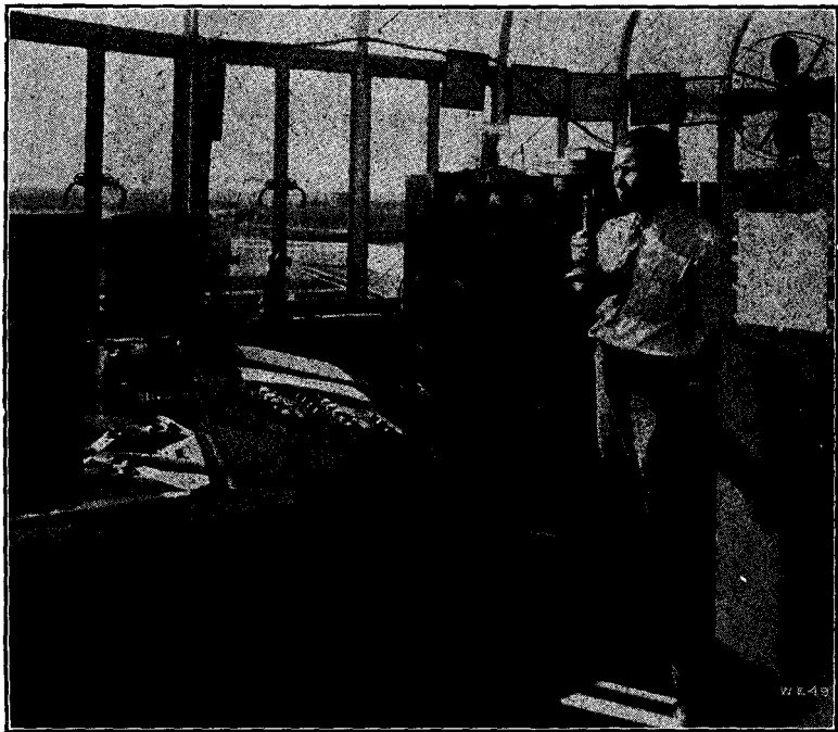
FIG. 3— Interior view of traffic control tower of modern airport. Dispatcher is directing the landing and take-off of aircraft by radio. The cabinet at the dispatcher's right is the airport's transmitter which puts his voice on the air. Other cabinets contain air line receivers, each one responding to the frequencies allotted to the respective lines. One receiver is utilized for reception of calls from itinerant flyers. On the desk are the loudspeakers working with the receivers and controls for lighting at the field, etc. (Courtesy Western Electric Co. Inc.)
