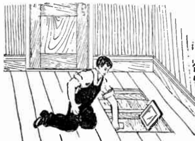
Fig. 7,280.—Method of exploring between floor and ceiling with flash lamp and mirror.
