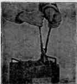
FIG. 6,334.—Battery repairs 34. Sometimes the bottom cover will not fit properly over the element. By using a pair of pliers in the manner illustrated, it will be an easy matter to locate the centers.
