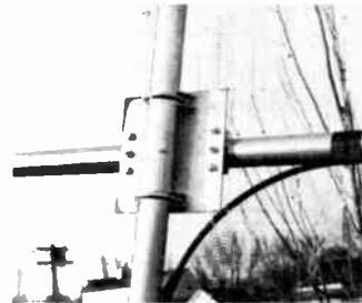
Fig. 14-55—The boom can be tied to the mast with muffer clamps and a steel plate. The coaxial line from the driven element is taped to the boom and mast.
