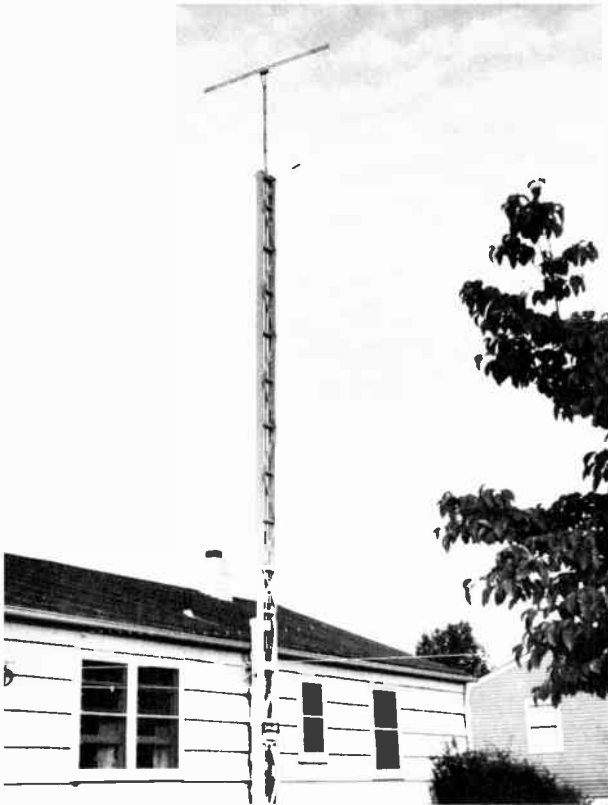
Fig. 21-57 — While guys are not normally required for the homemade tower, they provide an extra measure of protection against high winds. An inverted V can serve here as two of the guy lines.
