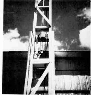
Fig. 21-67 — This close-up shows the rotor and cable installations. A double 2 X 4 is used as the base support for the rotator.
