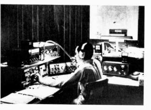
This modern amateur radio station is equipped for use in the hf bands. The gear is neatly arranged to provide the operator (K1ZND) with easy access to the various units. The foundation is made from plywood fashioned in the form of a console. The station belongs to K1THQ.
