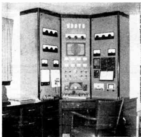
This neat "built-in" installation features separate finals and exciters for each band, along with room for receiver, frequency meter, oscilloscope, Q multiplier and v.h.f. converter. All units are mounted on the three large panels; the panels are hinged at the bottom so that they can be lowered for service work on the individual units. A common power supply is used, and band-changing consists of turning on the filaments in the desired r.f. section. (W9OYO, Sturgeon Bay, Wisc.)
