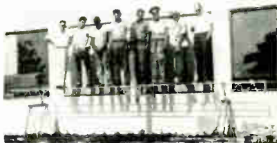
8-men (1200 lbs) test the strength of a C-10 section placed 15 feet between horses.
