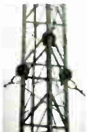
Typical Coupling and Guy Point
