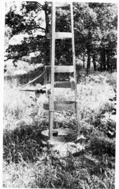
Fig. 63 — This photo shows the tapered base section with its winch.
