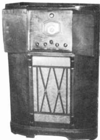
MODEL C-13-2 13 TUBES, 140KC-60MC 1935
