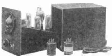
◇ RADIO ENGINEERING LAB'S, INC. ALL-PURPOSE RECEIVER 11-1000 METERS 4 TUBES $36.70 MAY 1931
