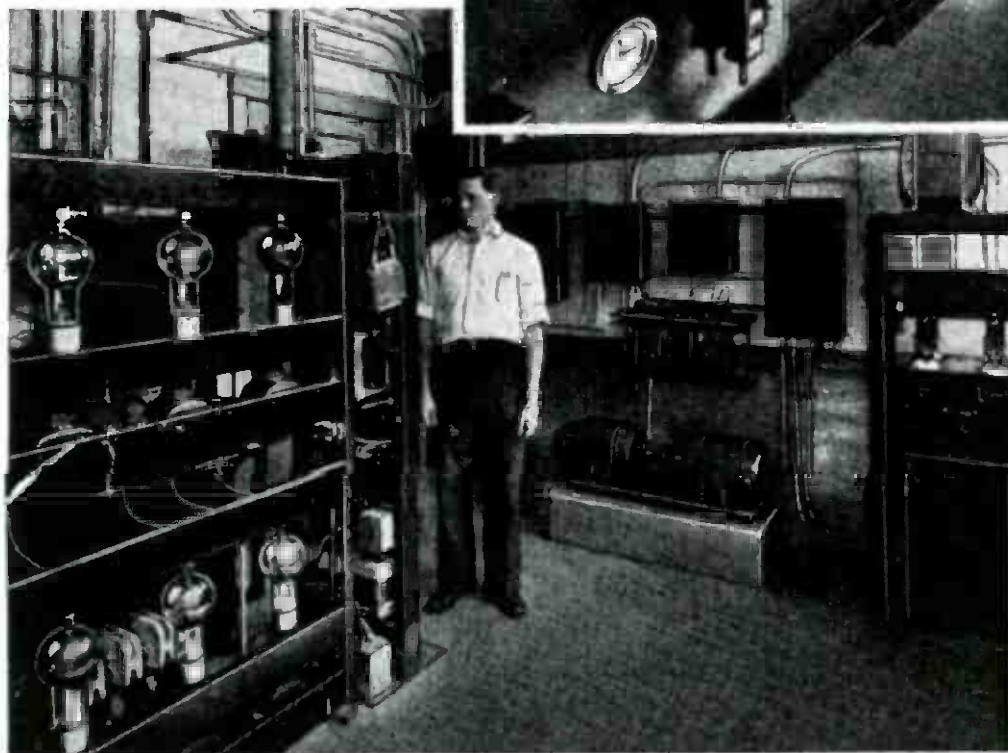
Photo above shows the 10 K. W. short-wave transmitting station operating on the well-known call letters W8XAL. This station has been received in all parts of the world and has entertained listeners as far away as New Zealand and Australia. The photo at the left shows the power equipment of W8XAL.
