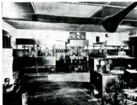
Illustration shows interior of Station KFKX at Hastings
