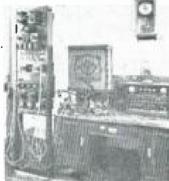
Amplificadores e controle Amplifiers and control room
