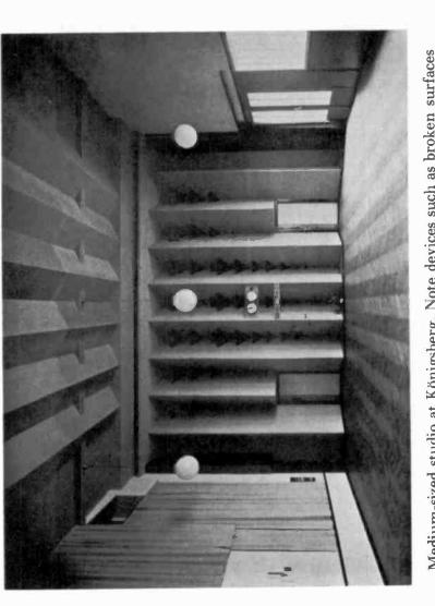
Medium-sized studio at Königsberg. Note devices such as broken surfaces of walls and ceiling and curtains for absorbing sound.
