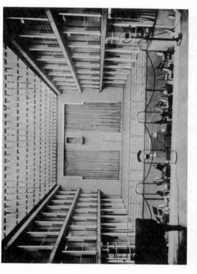
Large studio at Hamburg: Acoustic control by means of sliding walls, adjustable
