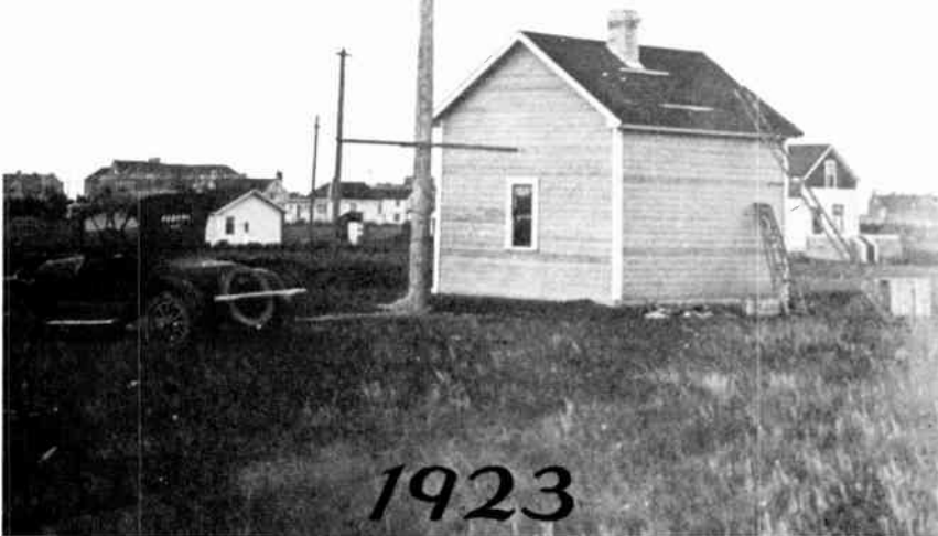
Typical radio transmitting building of the period. BROADCASTER MAGAZINE
