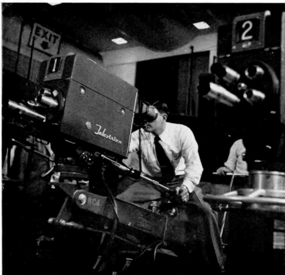
Here is the dolly camera, a kind of roaming reporter in the studio. Its huge bulk is pushed around by a "dolly man" at command of the cameraman, with whom he is connected by a complete telephone system.
