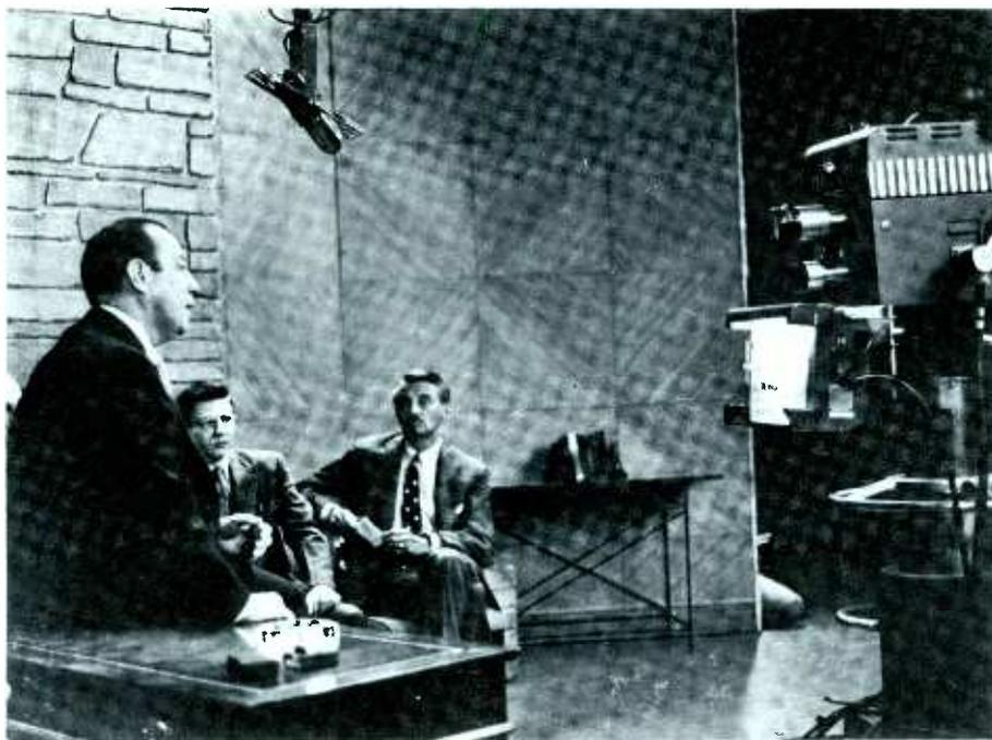
The TelePromptTer in use during a live performance. Note the RCA 77-DX microphone overhead. (Courtesy TelePromptTer Corporation)
