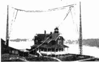
Lighthouse at Sea Girt, N. J., equipped for powerful transmission of compass signals and acting as a radio guide in the air and on the sea.
