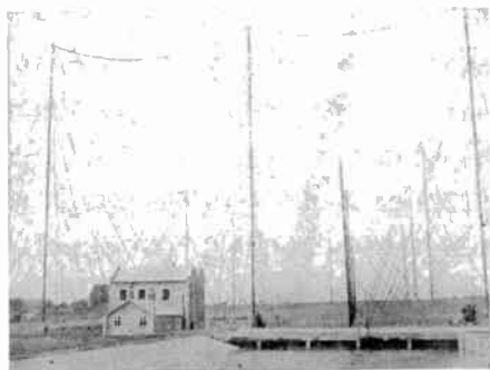
Part of the antennae at Seafield, England, used as a central radio-control station for India, Australia and all the most distant parts of the British empire. The arc system is used for transmission.
