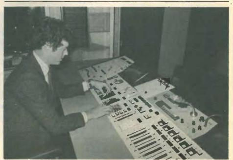
Studios 7 and 8 at BBC Television Centre are now being lit by a microprocessorcontrolled system developed by Thornlite in collaboration with the BBC's Capital Projects Department. The unit can control up to 500 studio lights and use nine Motorola 68000 microprocessors.
