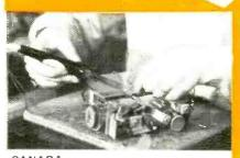
CANADA Ersin Multicore 5 Core Solder being used to solder Philco Auto Radios at the Philco factory, Don Mills, Ontario, Canada.
