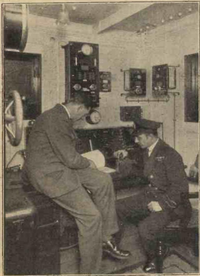
The latest liner of the P. and O. Company, the s.s. "Ranpura," is well equipped with wireless gear. This photograph shows the interior of the wireless cabin. The operator is seen adjusting a wavemeter.
