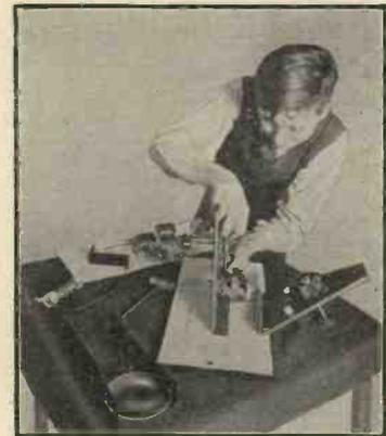
Showing the mounting of the motor to upright and fixing to the base board. Note the second upright has the bend facing inward, which is not apparent on the template.
