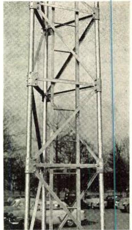
Heavy cross-bracing minimizes twist
