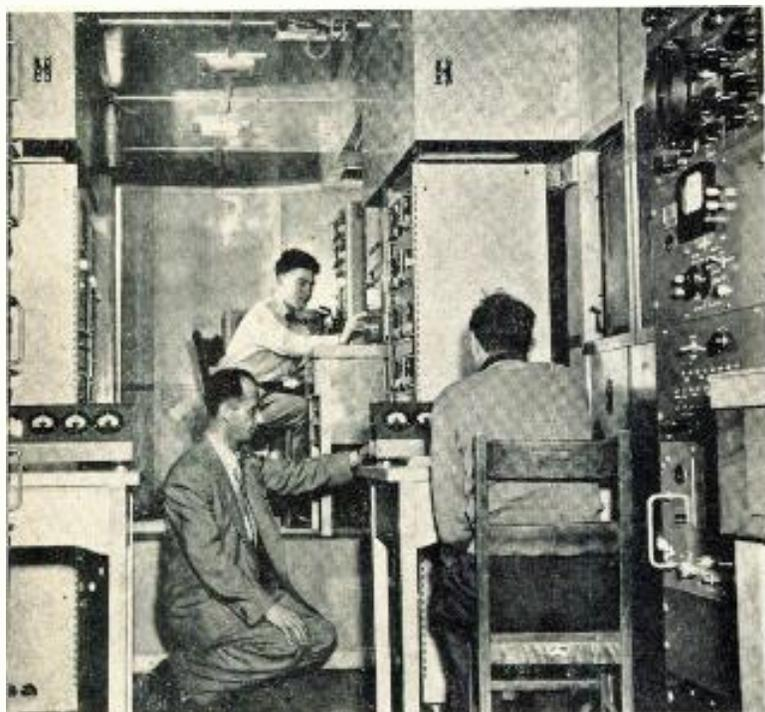
Radio telemetry has found still another application. At the jet airplane plant of A. V. Roe Canada Ltd, engineers and aerodynamists are now flight-testing their aircraft from a trailer-mounted telemetering pickup station which may be located as much as a 100 mi. from the testing area. The massive electronic receiving-recording apparatus inside the trailer is capable of recording 67 separate items of data per sec. in the course of the test flight.
