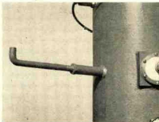
**SIMPLIFIED DESIGN** for antenna bay accessibility! This pole step with boss welded to bay facilitates beacon light maintenance or adjustments. Also useful as a twist lever for bay rotation when contouring.
