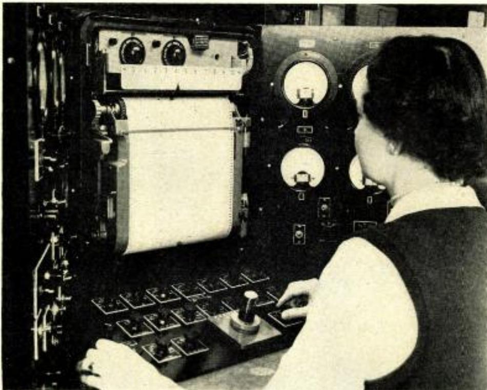
Fig. 1: Operator at controls of curve-tracer set observes tube characteristic curves being recorded
