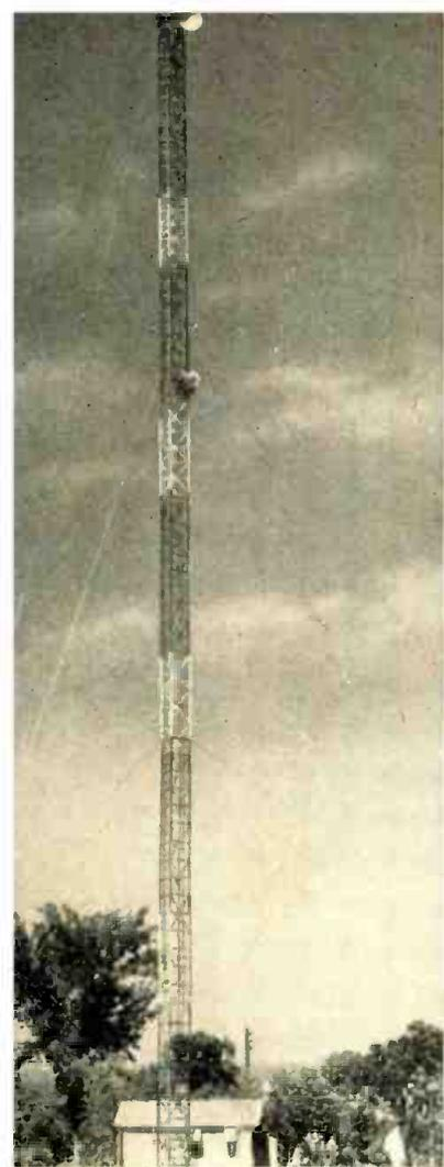
**RCA Microwave radio relay installation at High Ridge, Mo. Towers are rugged, designed to withstand 100-mph winds under severe icing conditions.**
