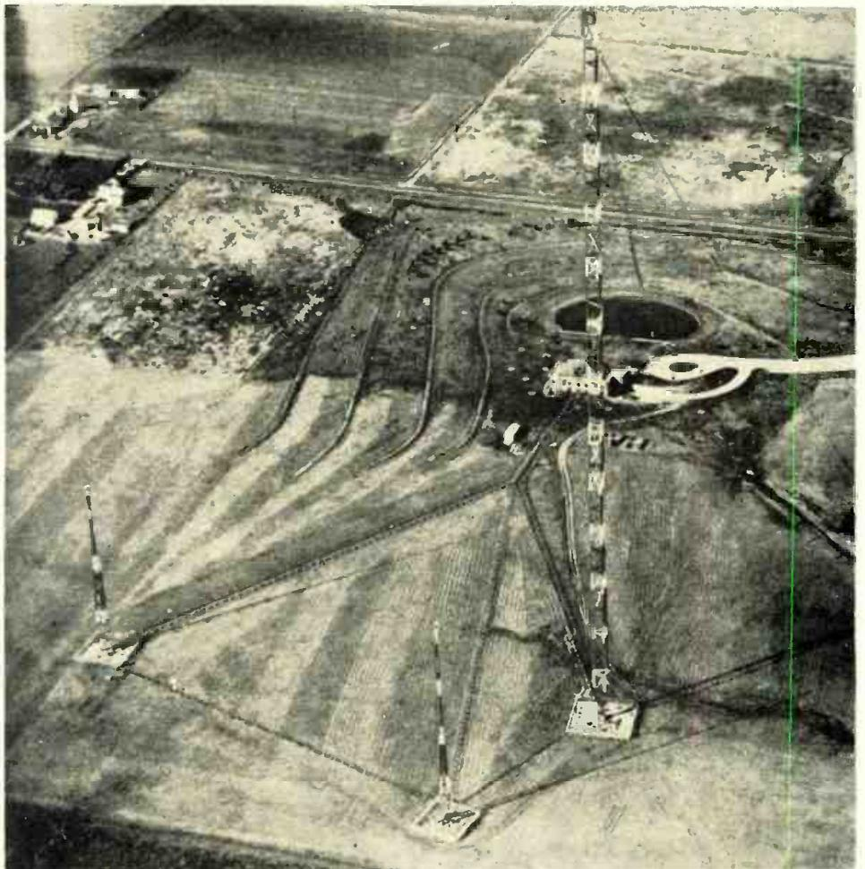
Fig. 2: Three-tower directional antenna system of station WKY, Oklahoma City, Okla.
