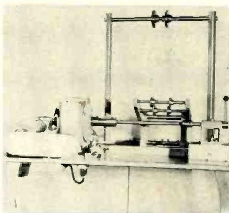
to 10 in. in length and 16 in. in diameter. Wire sizes are from 5 to 18 A.W.G. Winding speed is 50 to 85 rpm. A special 3/4 h.p. variable speed motor operates on 115/230 v., 60 cps, single phase. Geo. Stevens Mfg. Co., Inc., Pulaski Rd. at Peterson, Chicago 30, Ill.—TELE-TECH & ELECTRONIC INDUSTRIES.
