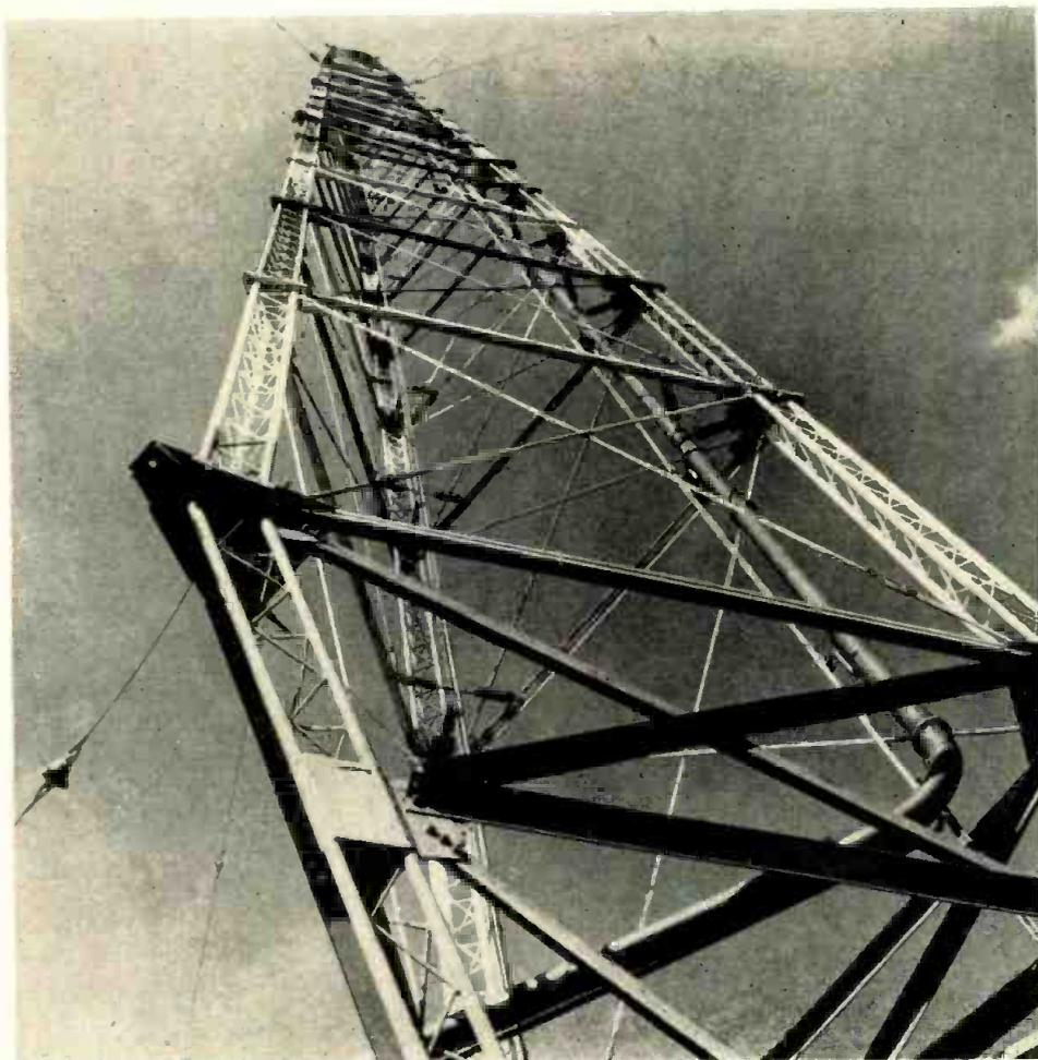
Fig. 3: Base view of WKY's Franklin antenna shows lines feeding TV and FM radiators at top
