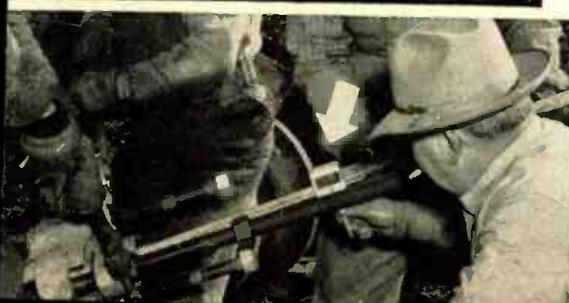
Invar measuring rule, an exclusive Blaw-Knox feature, is used to determine correct initial tension in the factory pre-stressed guys. Erectors use the rule when putting up the tower and can easily duplicate correct tension determined in the factory tests—thereby eliminating any guess work in the field erection.
