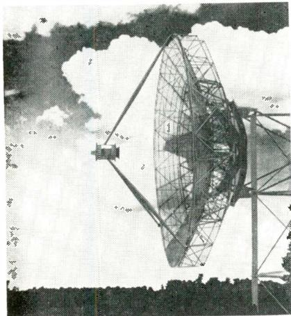
lation procedures, and economy of transportation. Reflector diameter is 28 feet. Focal length is 10.5 feet. Weight is 1,575 pounds. Wind load rating is 30 psf. Plane and bi-polar feeds are available for any frequency band in the range from 400 MC to 2700 MC. Andrew Corporation, 363 East 75th Street, Chicago, Illinois.
