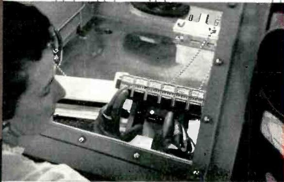
Contamination is eliminated. Baking, surface treatment, electrical testing and package welding are all conducted in dry-boxes at a dewpoint temperature below  $-90^{\circ}\text{F}$ .
