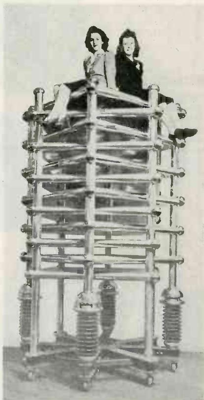
FEDERAL'S 200,000 volt 2500 mmf phantom antenna capacitor built entirely of non-critical materials
