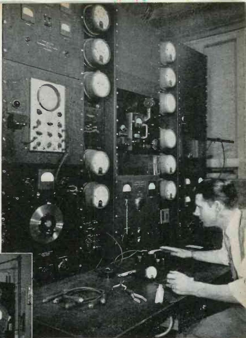
▲ MEASURING characteristics of a special instrument in the completely isolated high-frequency cage
