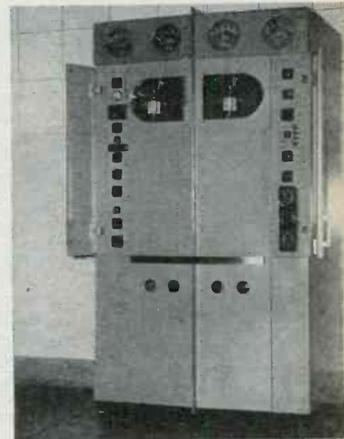
COVERING the county, transmitter for AM is a 1 kw Western Electric
