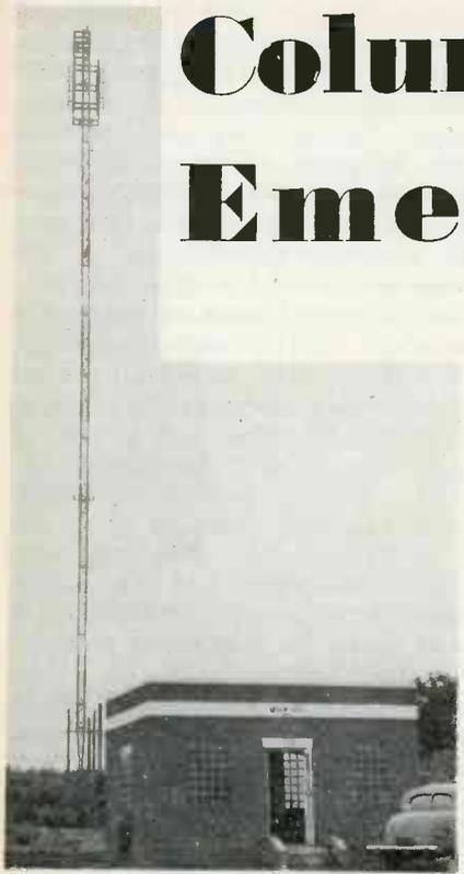
RECEIVING antenna is mounted on 200 ft. pole above another antenna
