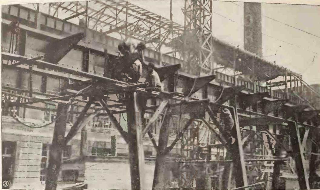
Building the Trestle Work for New Coal Conveyor to New Power Plant.
