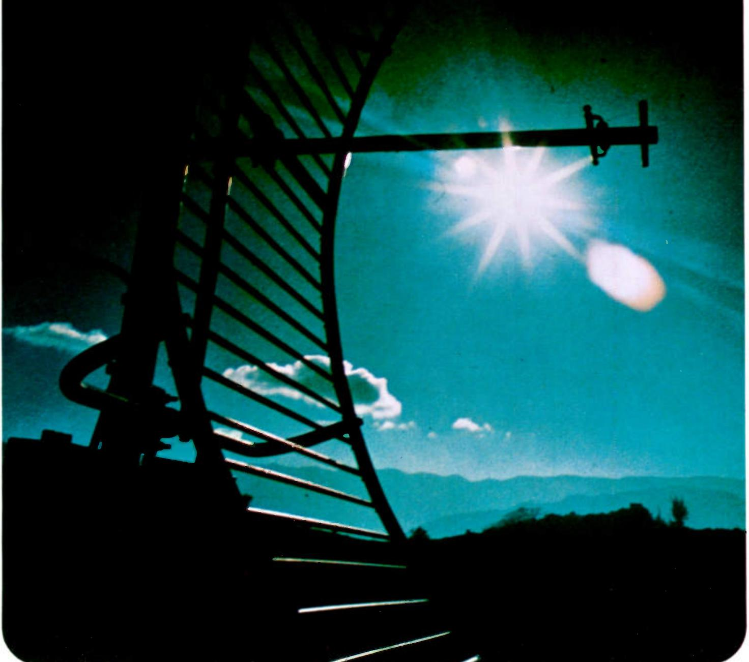
Shown above is a UHF parabolic section receiving channel 44 from San Francisco. It is located at Almaden, one of five head-ends currently bringing 20 channels to San Jose, California.
