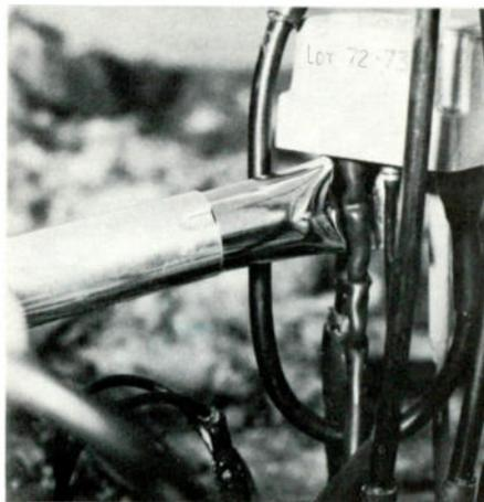
*500 watt electric heat gun putting out 500 F. is used to make splice cover in tight quarters at this house-drop from tap. Tape wraps would be difficult and time-consuming here.*
