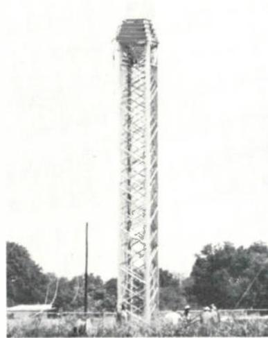
Stacked sections are pulled upright by tower guy wire. Rising sections pull remaining guys into place. No extra equipment required.
