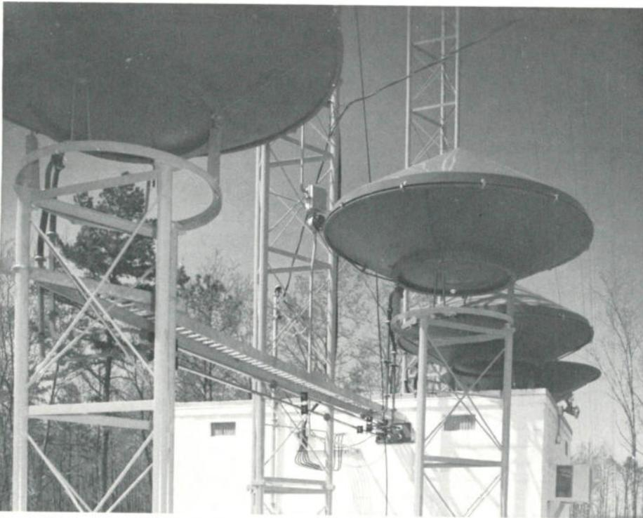
Figure 6. Milmay's cross-polarized, dual-feed transmitting antennas.
