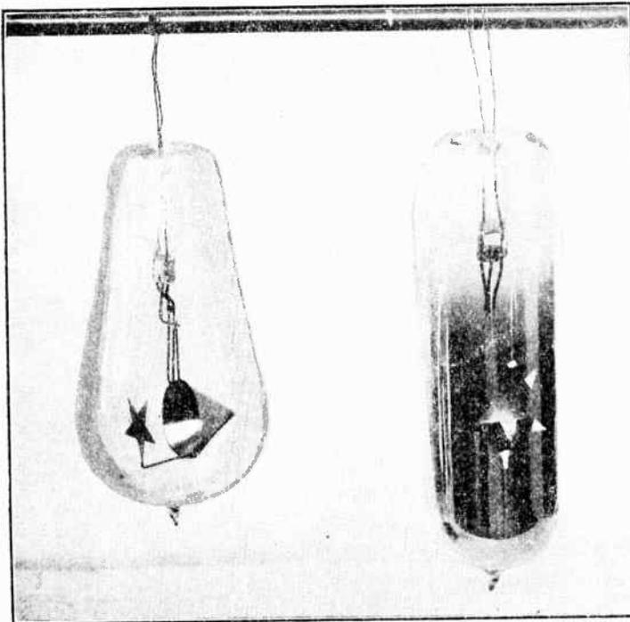
The evaporated gold from a gold-plated tungsten filament, in the experiment illustrated above, casts a marked shadow on the walls of the vacuum tube when a design is interposed, showing that the molecules of the evaporated substance travel in straight lines in high vacua.
