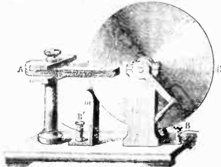
The modern generator is the industrial outgrowth of the simple experiment illustrated above. The permanent magnets induce electromotive force in the metal disc rotating between its poles.
