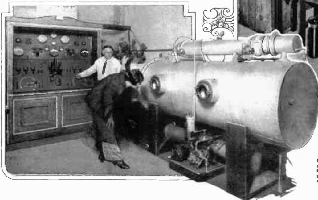
Electricity in the service of the embalmer is illustrated at the left. The dead body, placed inside the large retort, becomes dehydrated by electrically produced heat and the electrolytic action of a current passing through the body.
