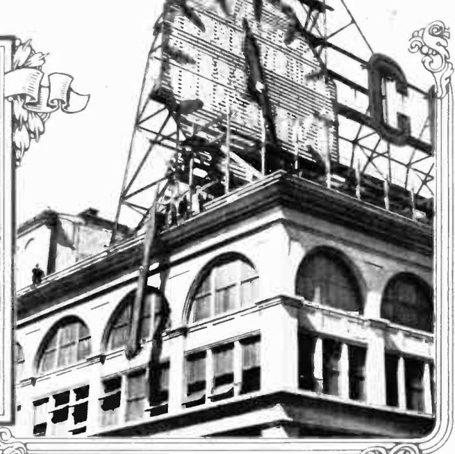
The picture above shows the hoisting of the hour hand of the huge clock being erected on the roof of the Colgate factory in Jersey City. This colossal clock, with its movement weighing four tons and run by a small one-quarter horsepower electric motor, is replacing the old clock shown at right. Note that in place of figures large rows of electric lights are used on the dial.
