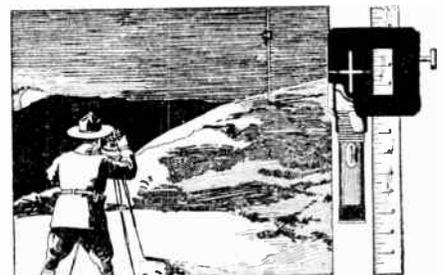
This target is for use on a leveler's rod. An electric flashlight is mounted on the rod, giving a luminous target upon which the leveler trains his instrument for reading the levels in the usual manner. Thus the device may be used in dark places.
