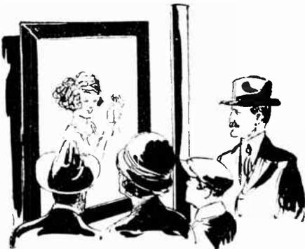
By analyzing an image into elementary portions and modulating a carrier wave in accordance with the space and intensity characteristics of each portion the image is transmitted by radio to the receiving station. A combination of photoelectric cells and electron streams makes the transmission possible. The illustration shows the receiving end of the apparatus.
