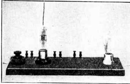
This spectacular experiment illustrates grid control in a striking fashion. An incandescent lamp illuminated by the plate current of a radiotron was extinguished by the approach of a charged piece of insulating material to the upright wire connected to the grid.
