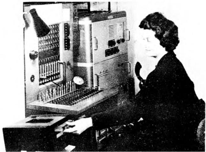
will play continuously until removed. Although fully equipped for playing tapes through internal speakers, the Playdeck is designed for connection to external audio and PA networks. One of its most obvious uses is to provide a non-stop supply of 'canned' music in factories, supermarkets and canteens, where indeed it has already proved popular. **Manufacturer: Magneta (B.V.C.) Limited, Ackmar Works, Parsons Green Lane, London, N.W.6.**
