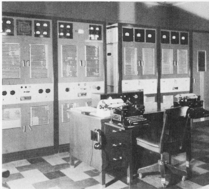
WTAG's five kilowatt transmitter is the latest development in broadcast transmission. Within these shuttered cabinets the electrical impulse from the microphone at the studio meets the radio carrier wave, which originates at a crystal which must be kept at an exactly even temperature constantly. The "sound" wave is superimposed on the carrier wave, or radio wave, to be radiated from WTAG's triple towers to your receiver.
