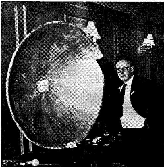
G3OAD, Dudley, Worcs., has contrived a 4ft. diameter dish aerial fabricated from fibre-glass and, presumably, covered with aluminium foil (details are not given). The important thing is the shape of the dish and the positioning of the feed point. We are informed that G3OAD can supply the details.
