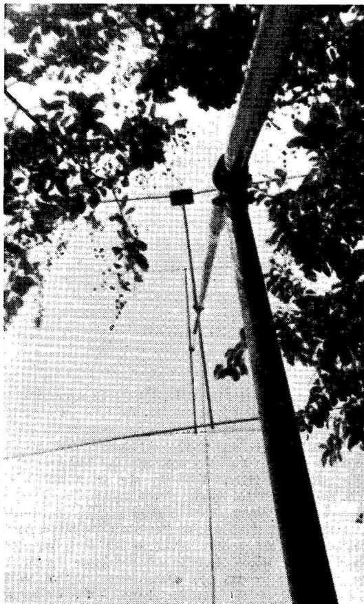
Looking up towards the fulcrum point, about which the clevis moves, as the mast comes up to the vertical. At this stage in the erection process the hauling up is quite easy, as the centre of gravity of the whole assembly is approaching the vertical.
