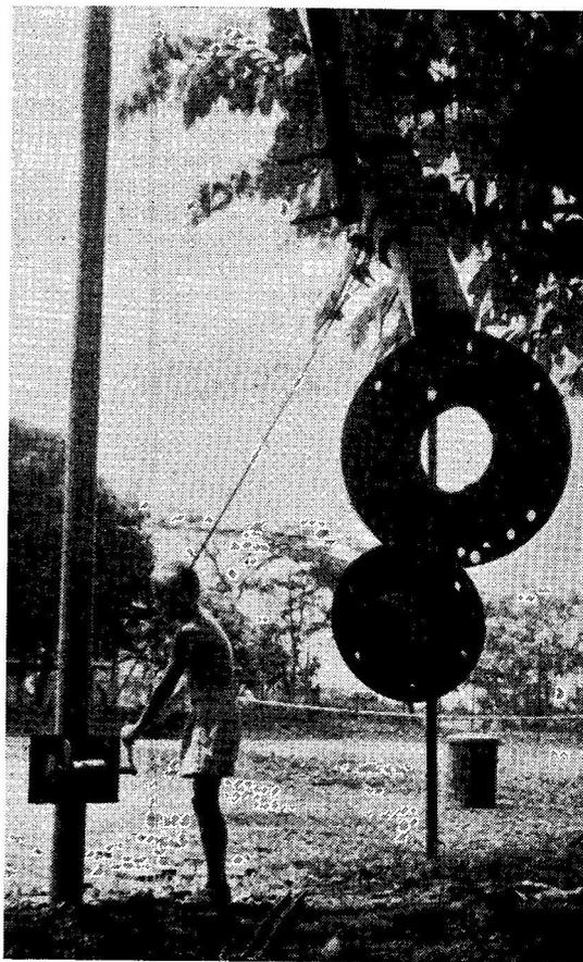
The heavy pieces of iron are hung on temporarily to counter-weight the mast, reducing the top-heavy weight to about 30-40 lbs.—making it possible for young 9LHX (Junior) to haul up Dad's 20-metre Quad on its 60-foot mast—see text.
