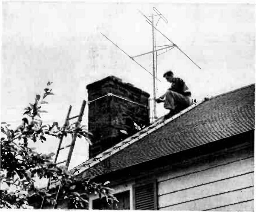
Fig. 5. Use of double-extension ladder and single ladder with roof hooks to get up to the chimney of a house safely for installing a television antenna. (RCA Victor photo)
