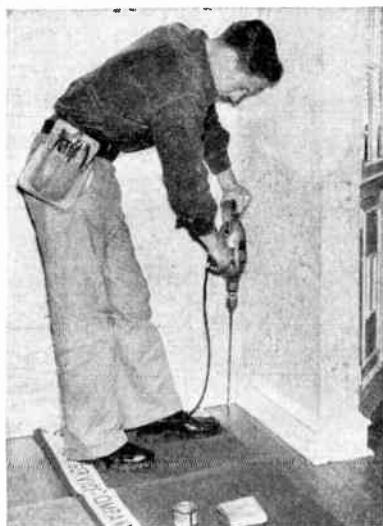
Fig. 11. Drilling a hole in the floor close to the wall behind the selected receiver location, for bringing up the transmission line from the basement. (RCA Victor photo)
